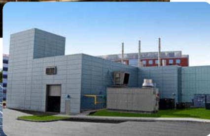
Princeton Hospital, NJ served by NRG Energy Center Princeton
