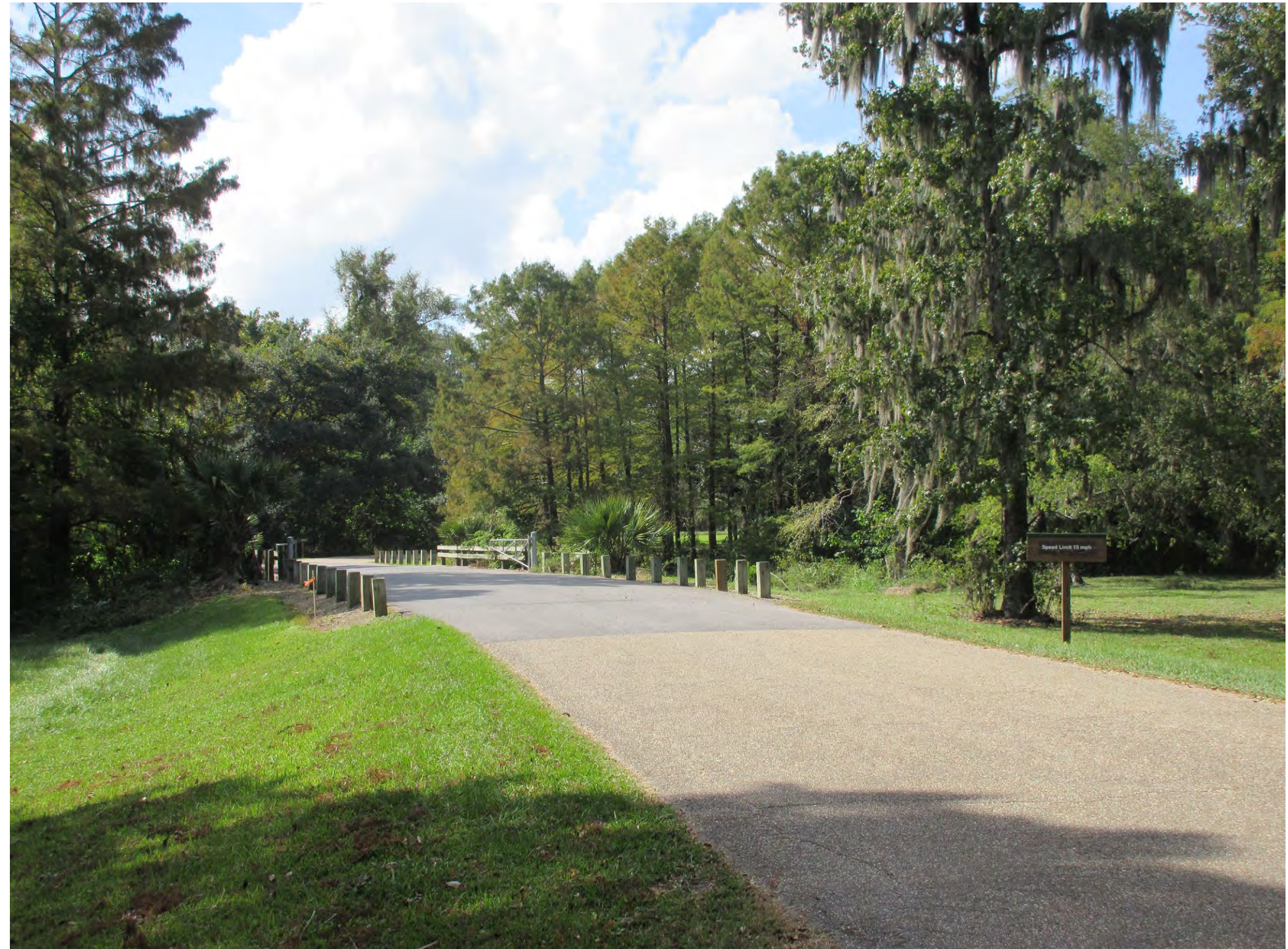
Figure 2.7 Existing Bridge to RLM, 2020
