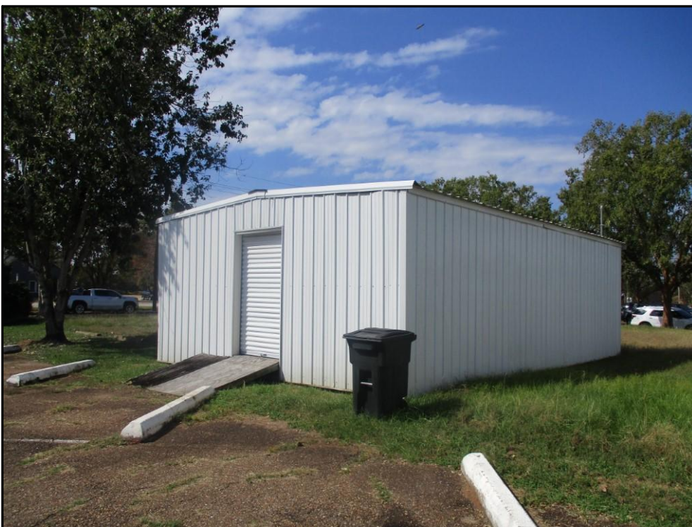
METAL BUILDING ON SITE
